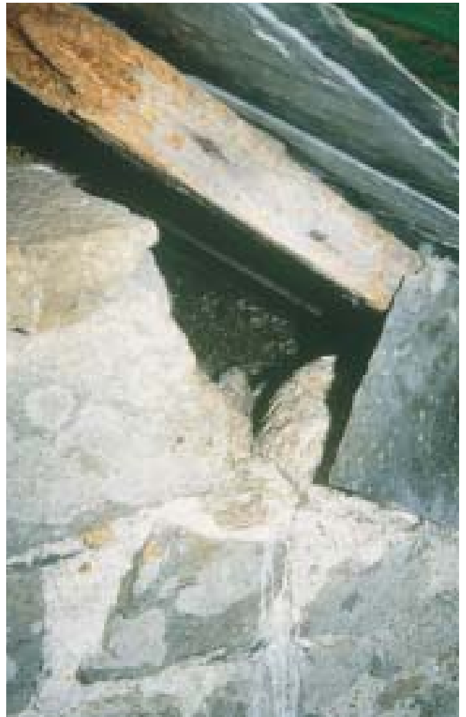
Picture 9 This cavity (note the debris and droppings) was accessible only from the outside of the site and could easily have been missed during a survey. David Ramsden
